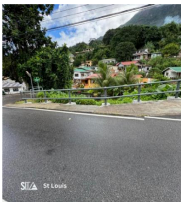
St Louis Installation of crash barriers “dan koko”
