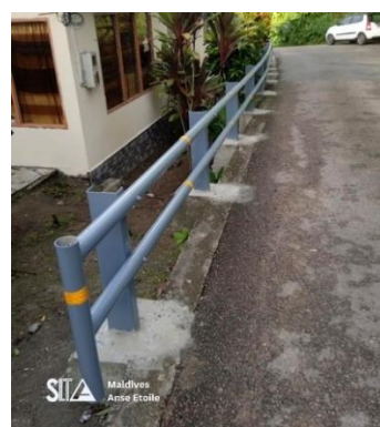
Anse Etoile Installation of crash barriers at Maldives
