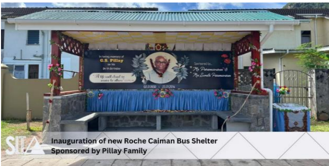
Donation by Pillay family/Designed and supervised by SLTA Construction of new bus stop at Roche Caiman
