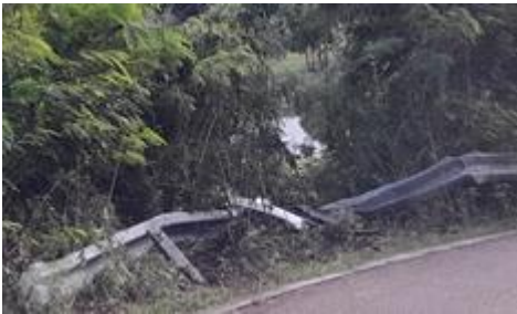
Maintenance work Repair of damaged crash barriers Cote D'Or Baie Ste Anne, Praslin
