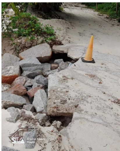
Coastal Protection – Anse La Blague Repair of the Anse La Blague road following coastal erosion
