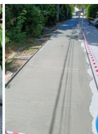
CAPEX Project Patching of damaged concrete road surface from Chateau St Cloud to La Passe La Digue
