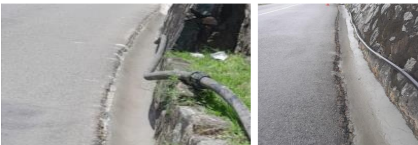
Anse Etoile Drainage improvement opposite Ma Constance Store
