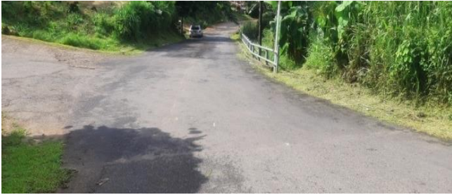
Anse Aux Pins Resurfacing of Caryole Bridge
