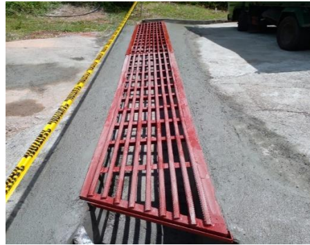
Port Gland Installation of steel grill
