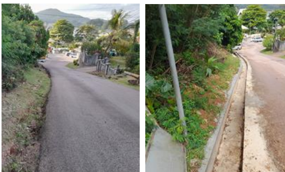
CAPEX Project Drain at Pointe Cabri Baie Ste Anne, Praslin
