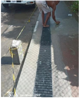
Les Mammelles Maintenance and repair of the drainage system
