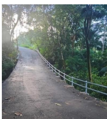
Au Cap Installation of crash barriers at St Roch
