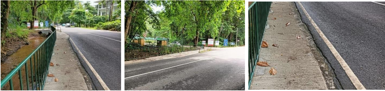
Beau Vallon Construction of footpath in the Boathouse area
