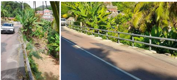
Maintenance work Installation of crash barrier Baie Ste Anne, Praslin
