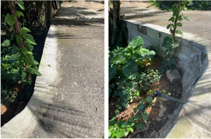
Mont Buxton Repair of La Poudriere road
