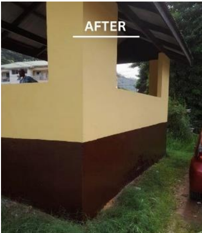
Cascade Maintenance of bus shelter at Talbot
