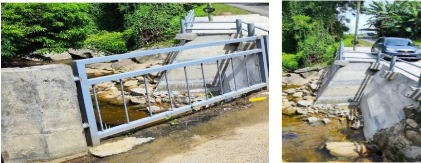
Bel Ombre Bridge renovation at Mt Simpson
