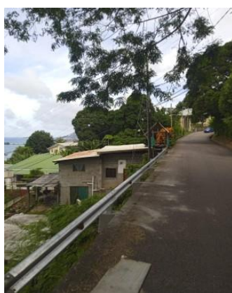
English River Installation of crash barriers at Union Vale
