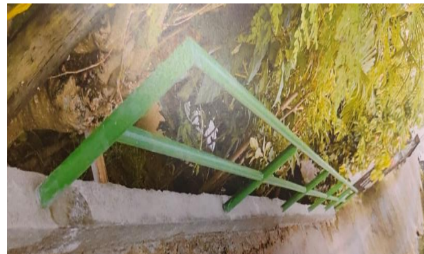
Plaisance Installation of crash barrier at La Louise
