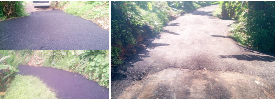
Anse Aux Pins Resurfacing of Land Bank road
