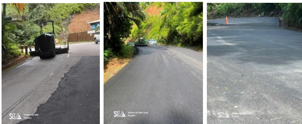
Planned project – Vallee de Mai road Resurfacing of the road
