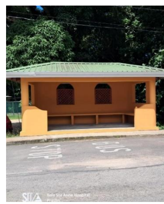
Maintenance work Maintenance of bus shelter at the hospital Baie Ste Anne, Praslin
