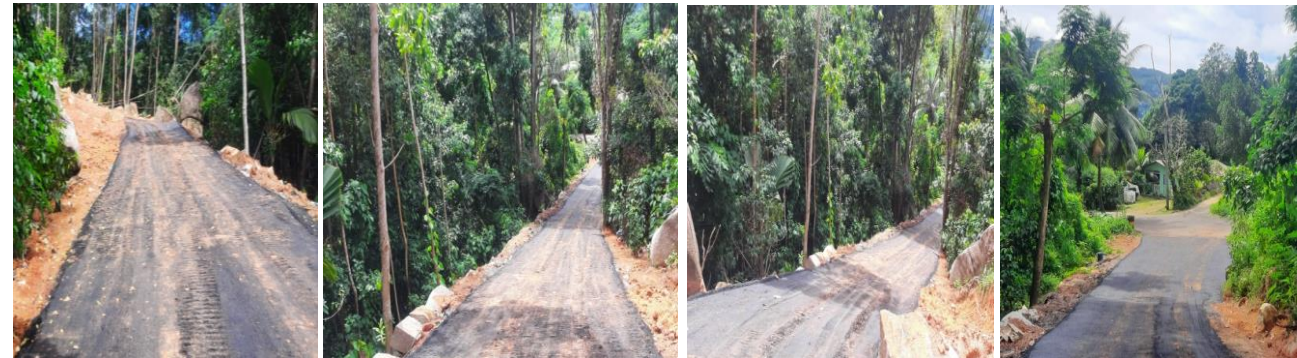
Anse Royale Resurfacing of "kot Rabbat" road
