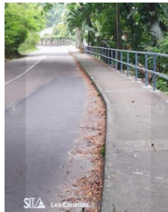
Les Canelles Maintenance of handrails
