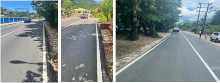
Anse Boileau Centre and edge lines were demarcated on the new road surface from Anse Boileau Clinic until Junction Anse Boileau, Mt Posee.
