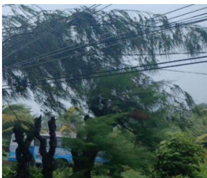
Emergency work - Disaster Event 3.1.24 Fallen branch over electrical lines Anse Kerlan, Praslin
