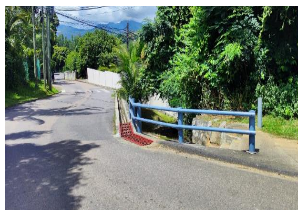
Anse Etoile Installation of crash barriers at Foyer de Nazareth La Gogue
