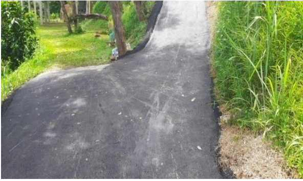
Bel Ombre Resurfacing of Doctor's Road
