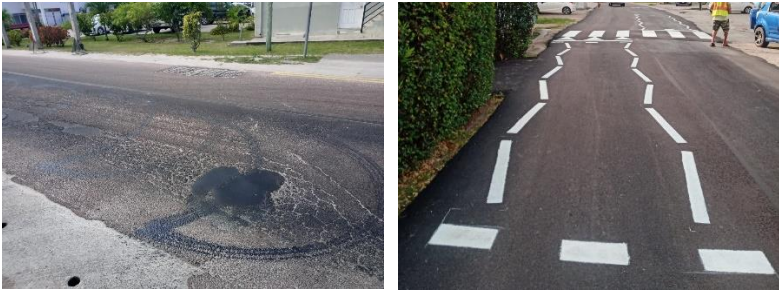
Planned project – Grand Anse Praslin main road Resurfacing of the existing asphalt main road to improve its condition
