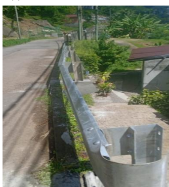
Bel Ombre Installation of crash barrier at Le Niolo
