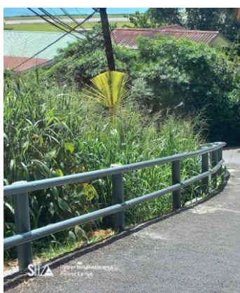
Pointe La rue Installation of crash barriers at Upper Rosabelle area
