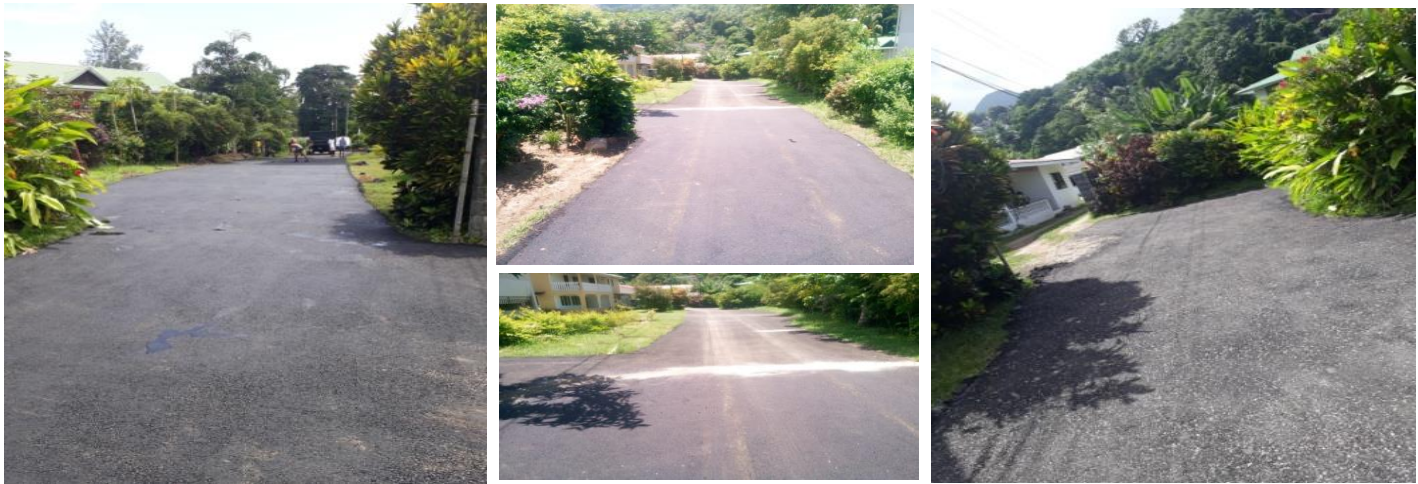
Anse Aux Pins Refurfacing of Chetty Flats road
