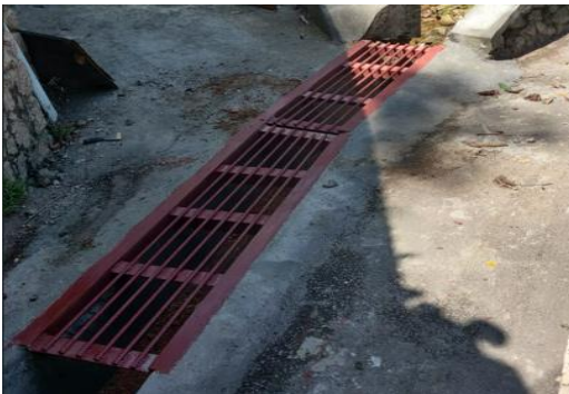
St Louis Repair of steel grill
