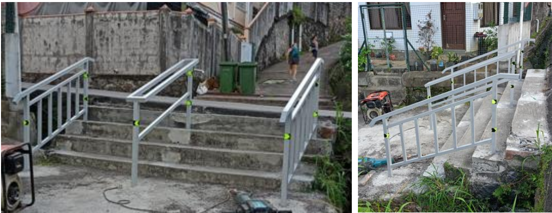
St Louis Installation of handrail
