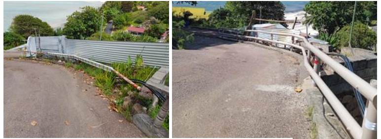
Maintenance work Installation of crash barrier at Au Cap Baie Ste Anne, Praslin
