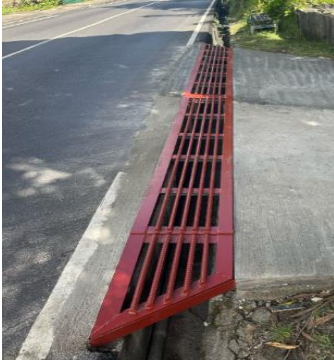
Beau Vallon Replacement of damaged grill
