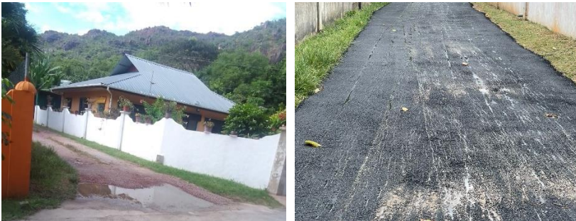
Planned project – Baie Ste Anne, Praslin Surfacing of earth road to improve its condition
