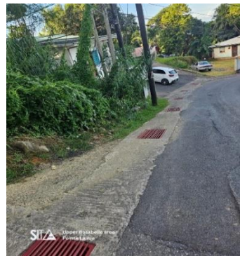
Pointe La rue Grills installed over the drainage system at Anse Francois
