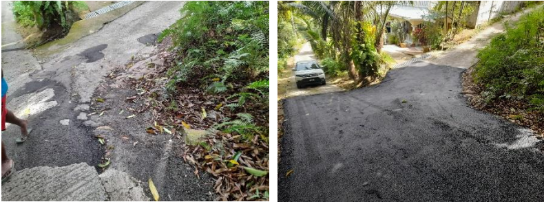
Planned project – Baie Ste Anne, Praslin Repair of the damaged Markham road by resurfacing the existing asphalt
