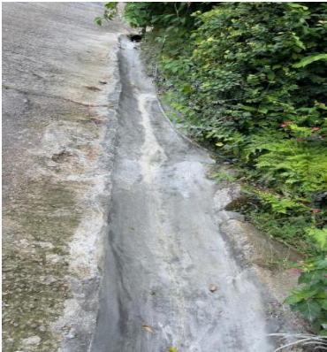
Plaisance Drainage improvement at Kan Frichaud
