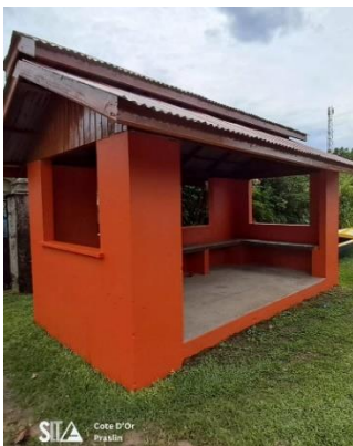
Maintenance work Maintenance of bus shelter at Cote D'Or, Praslin
