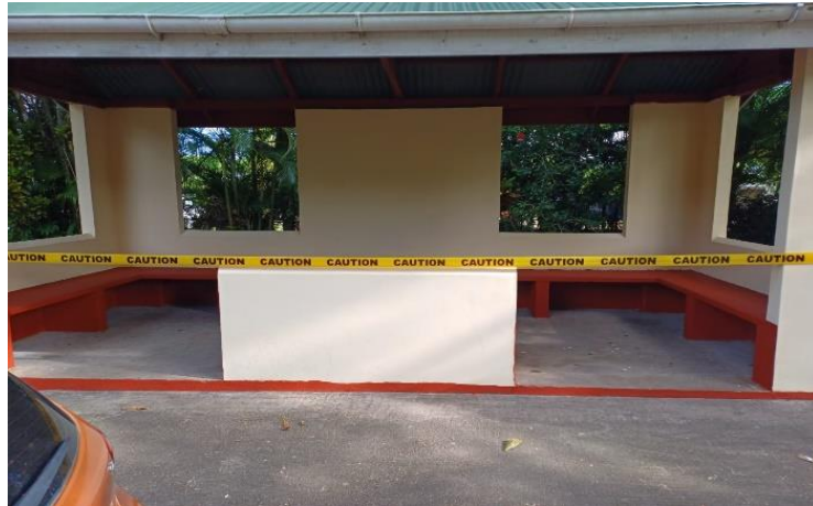
Anse Louis Maintenance of bus shelter
