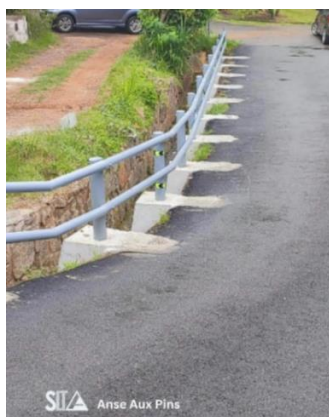
Anse Aux Pins Installation of crash barriers
