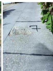
CAPEX Project Patching of damaged concrete road surface from Chateau St Cloud to La Passe La Digue
