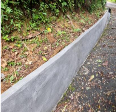
Anse Etoile Construction of collapsed drainage wall at Angar
