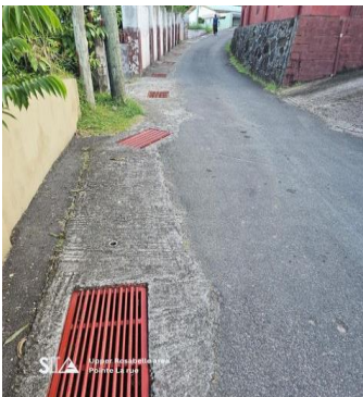
Pointe La rue Grills installed over the drainage system at Anse Francois
