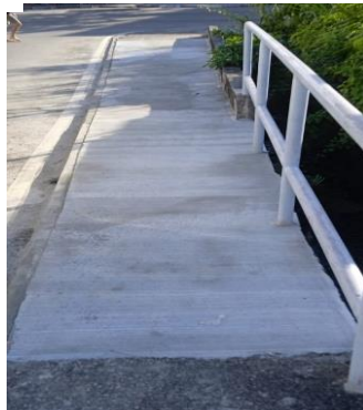
Plaisance Installation of crash barriers at Belvedere
