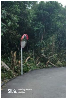
Au Cap Repair of traffic mirrors
