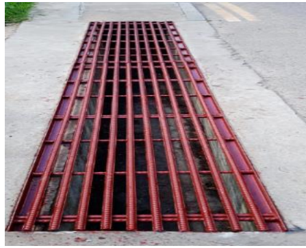
Anse Etoile Replacement of steel grill at Anse Etoile Fish
